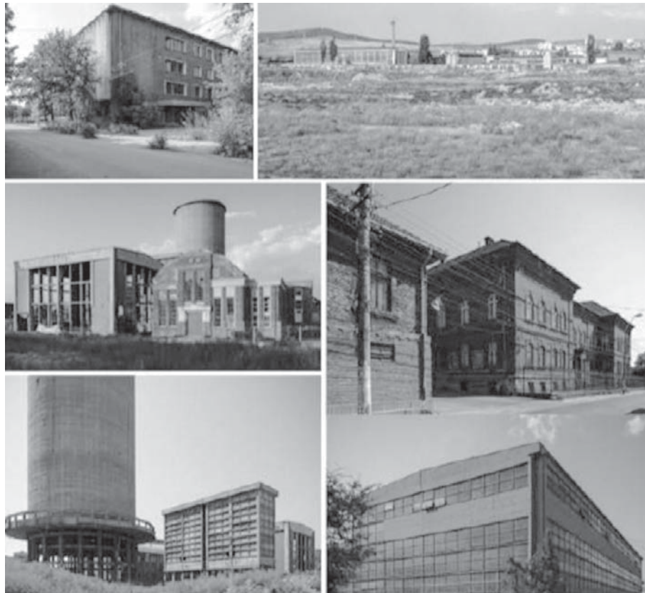
Fig. 5. Photographic survey of tangible traces of Hunedoara industrial territory. Source: Paolo Mazzo, July 2013
