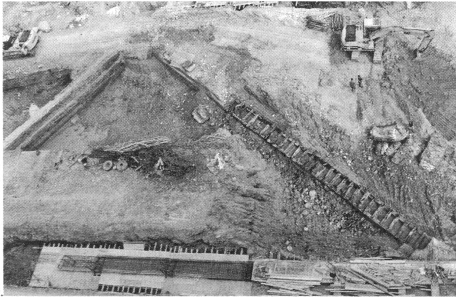
PLATE IV: 1 – The wooden substructure mounted on pillars in the southern half of Counterguard I (City Business Center, Building D); 2 – The wooden substructure directly on the yellow clay, in the northern half of Counterguard I (The 700 Square underground parking area).
