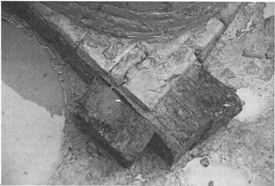
PLATE VI: 1 – The tip of Redan II, affected by the works of digging the foundation for a supporting pillar; 2 – Detail of the wooden structure underneath the foundation of the redan tip.
